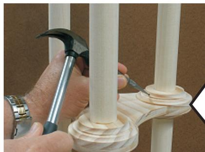
Drive in the nails and countersink with a nail punch. Fill the holes with a dab of wood filler. (fig. 4s)
