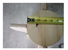
Create a layout line for screws like you did earlier with the table. Approximately 1" in from every edge put a 1 5/8" screw down into the legs.
