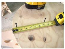
Put a crew in as shown above into the line you traced. Put one in at the 1" and 7" mark. 15/8" screws work great for this. Repeat on all four lines.
