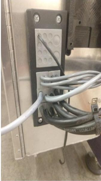
**LEFT:** For an Icotec cord fixture, remove the 3 bolts from the left side of the black fixture, and pull the side out. Remove one of the bottom gray squares, and run accessory cable into the control box, using one of the plugged holes in the gray square cable holder. Slide the gray square back in place, and reattach the left side to the fixture, making sure the cable reaches the driver.
