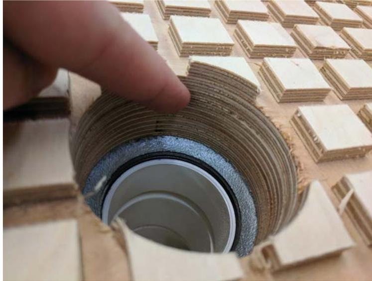
Once all the caulking is in place, install the spoil board in the locations shown.
