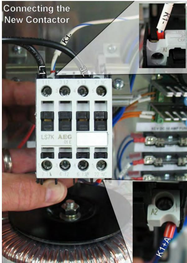
Locate the contactors and wires that came with the kit. The Blue/white wire (K1-) should be installed into the new contactor in position A1 located along the top and the Blue wire (K1+A) should be at position A2 on the bottom of new contactor.
