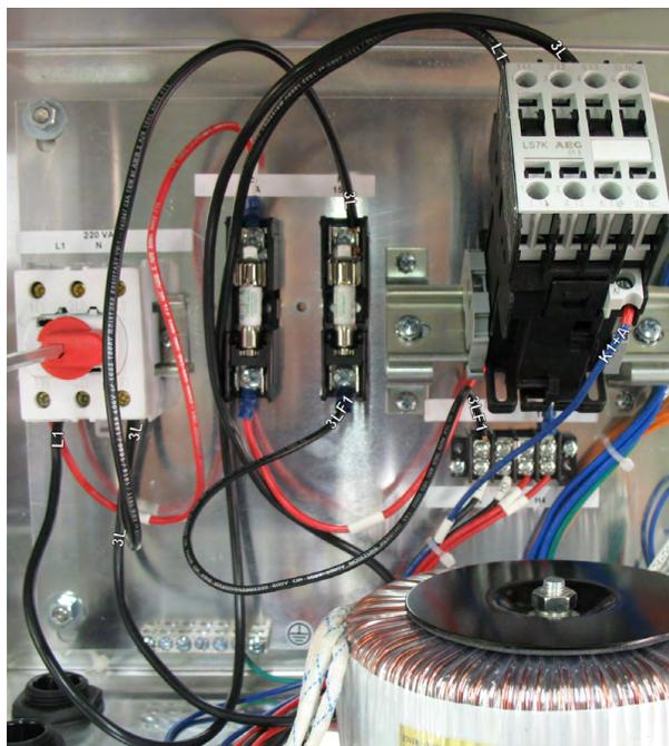
Take the loose end of the Black L1 wire from the contactor and wire into the main disconnect at position (2T1). This connection will be shared with a Red wire going to the top of the 1<sup>st</sup> fuse holder.
