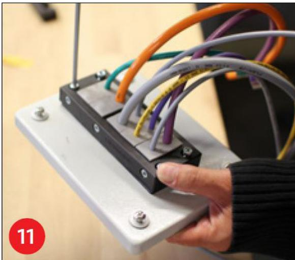
...and screw the cable entry frame to the control box.
