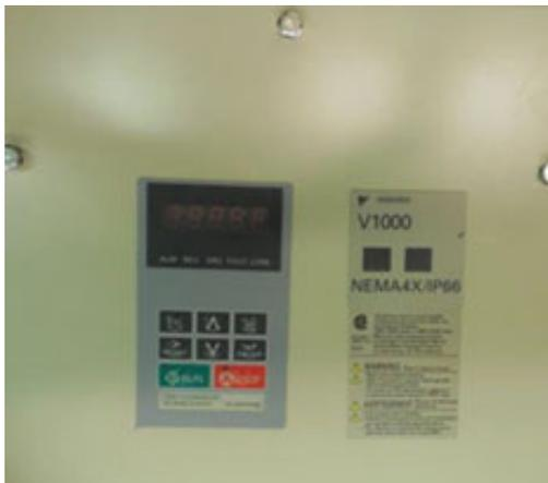
There are two main types of VFDs, a 10” model and a 16” model. These can be easily differentiated by their size and model numbers. Model numbers are found on the front of the VFD underneath the “RUN” and “STOP” buttons as shown on left.
